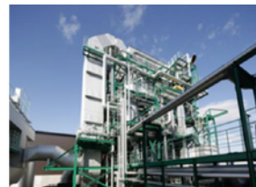
Biomass power plant
