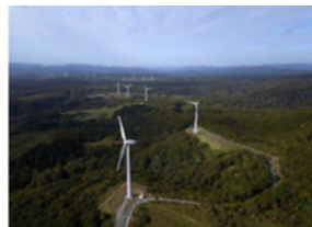
Wind power plant
